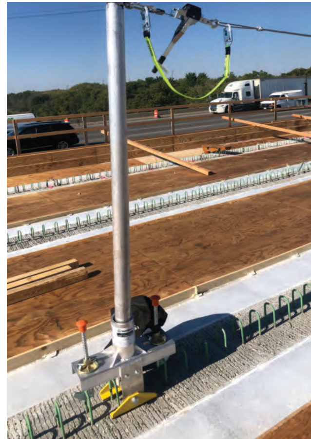
Intermediate Span Installation
